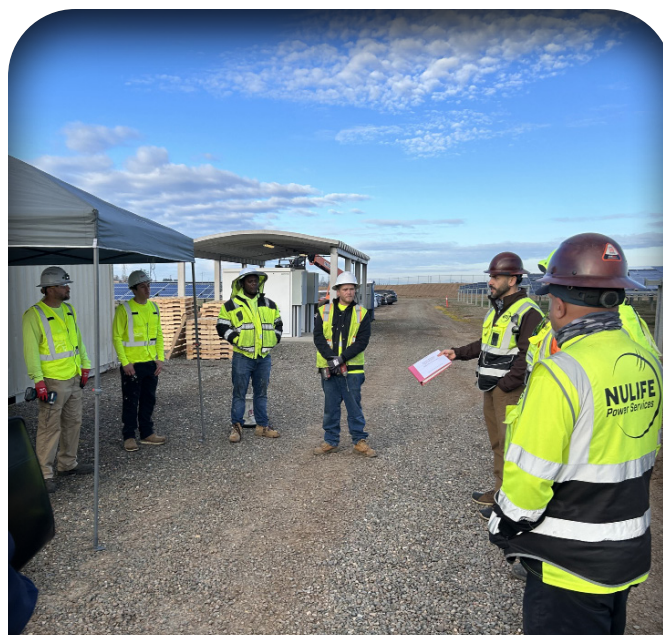
Figure 5. SSJID’s repowering contractor provided engineering and construction services and coordinated all field activities. (Credit: NuLife Power Services)
