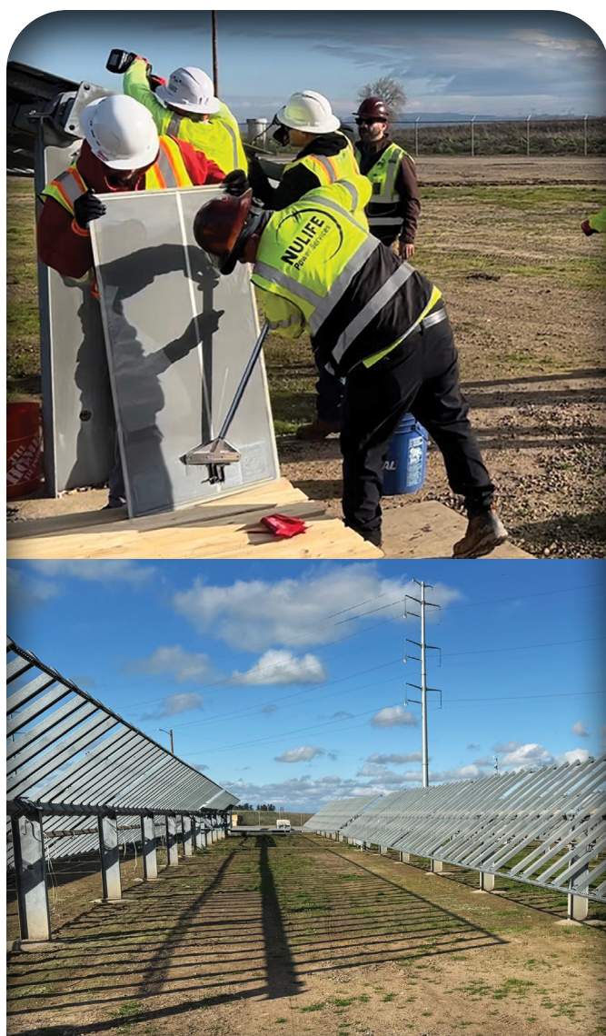
Figure 6. CdTe modules were processed according to First Solar's instructions, and tracking array frames were reused with a new module layout. (Credit: SSJID)
