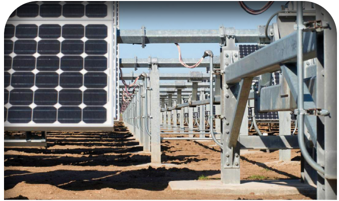
Figure 4. Replacement of legacy technology and reuse of industrial-grade support structures were foundational elements of the repowering plan. (Credit: SSJID)
